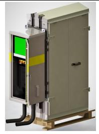
Install first four pairs of washers. Offer the **power annexe** up to the four bolts, when in place add the final pairs of washers and complete with **nyloc hex nuts**.
