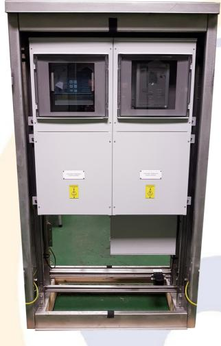
Adequate space below gland area to accommodate minimum bending radii of incoming cables.
