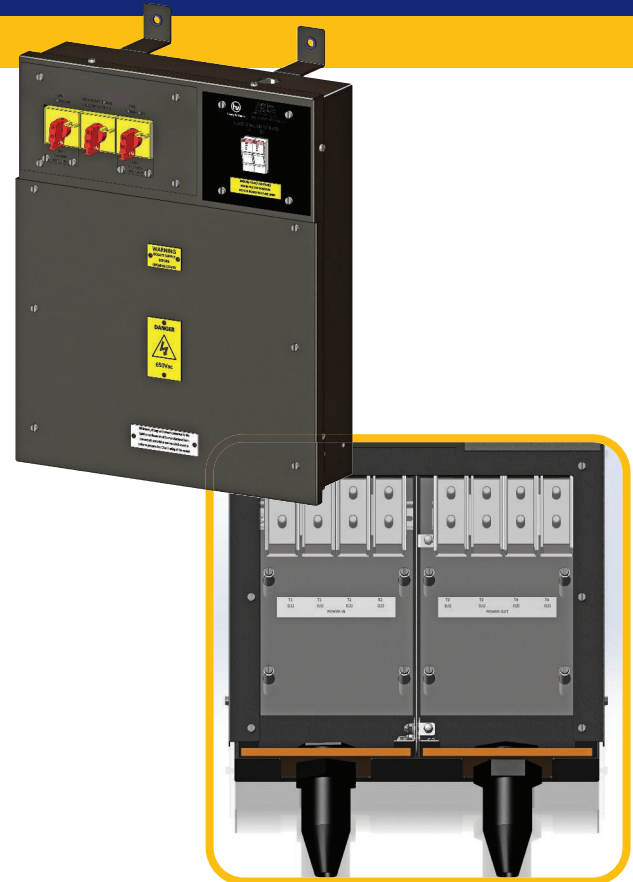
Main Terminal Arrangement
