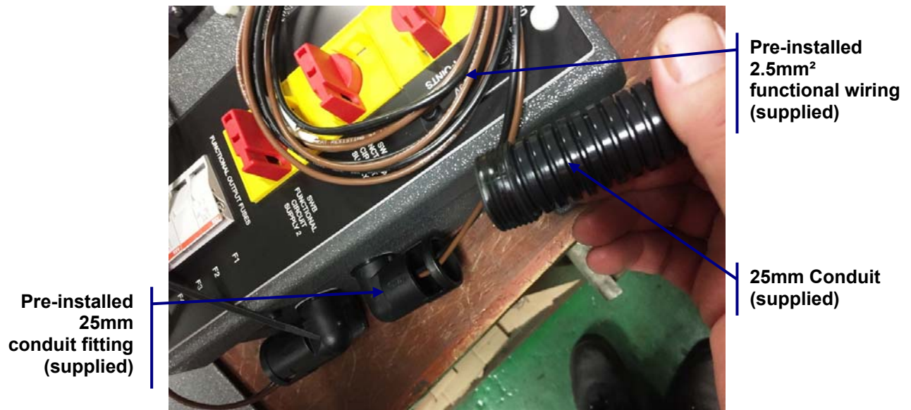
Figure 3: Functional Circuits/Transformer Wiring Outlets
