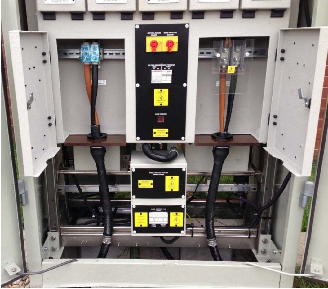
Figure 14: Final installation of terminated cables
