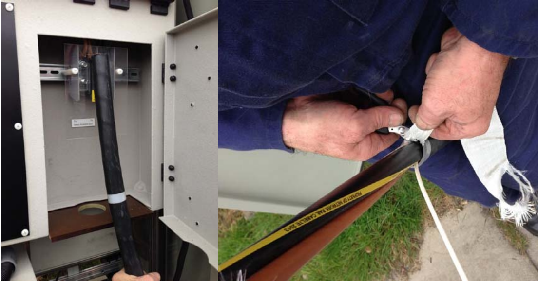
Figure 4: Measure & Strip Cable
