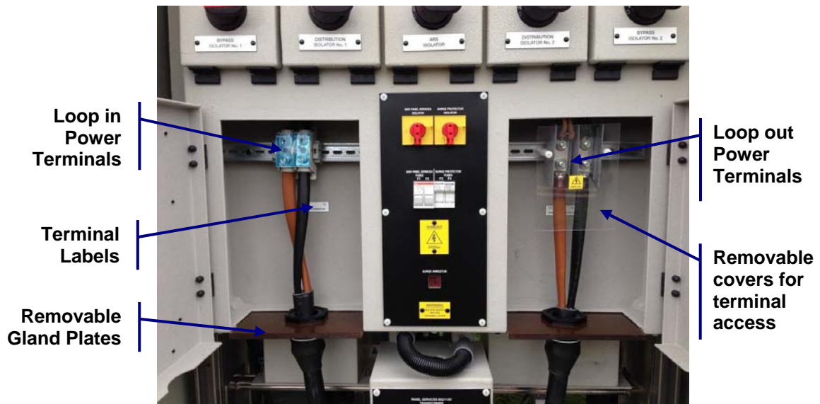
Figure 3: Power In/Out Terminal Arrangement
