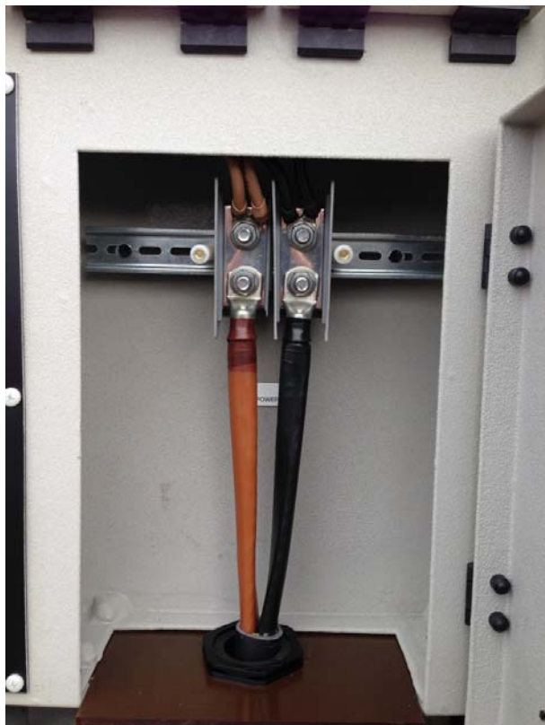
Figure 13: Tape crimps & terminate cable
