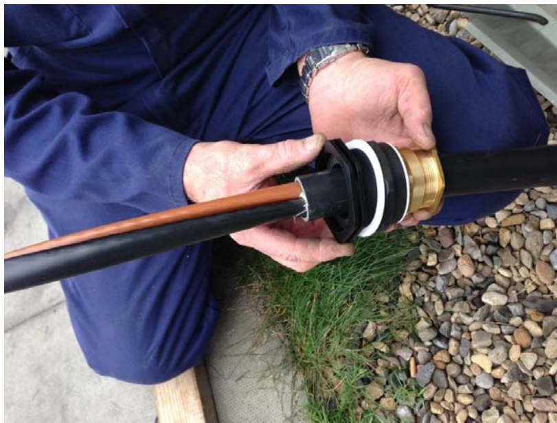
Figure 5: Fit Shroud followed by Gland onto Stripped Cable
