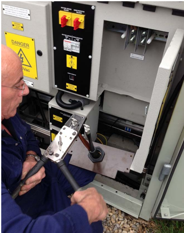
Figure 12: Crimping Cable Lugs
