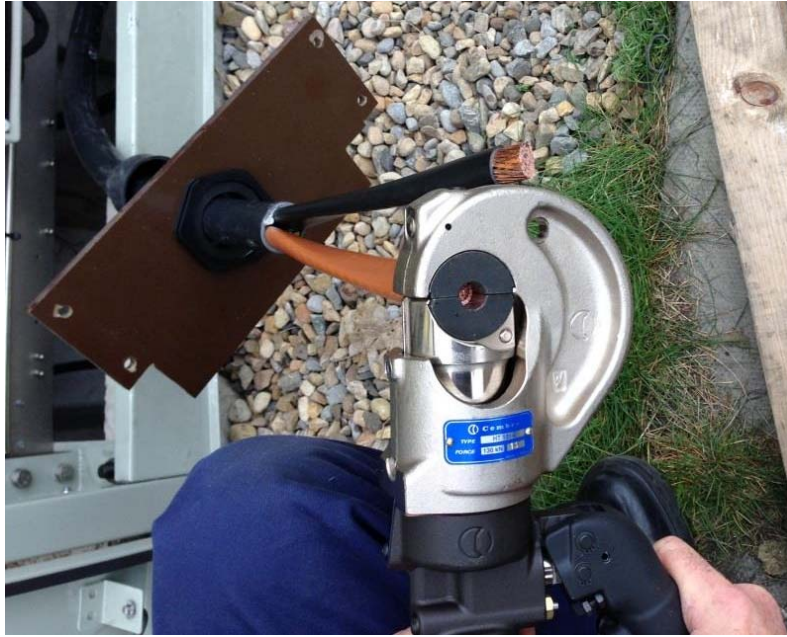
Figure 10: Rounding Cable ends using tool
