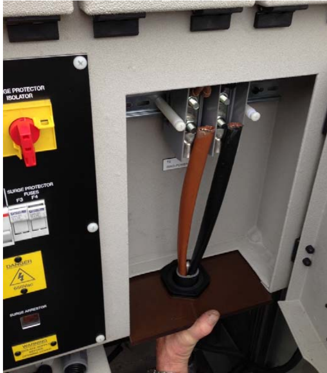
Figure 8: Cable length marked ready for cutting
