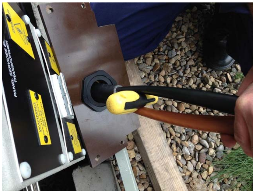
Figure 7: Forming Cable V shape
