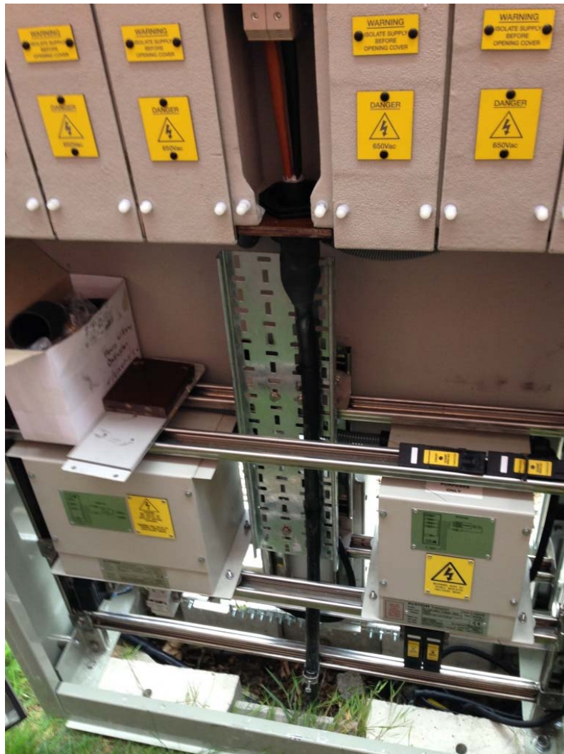
Figure 18: Secured External Loads Feed Cable
