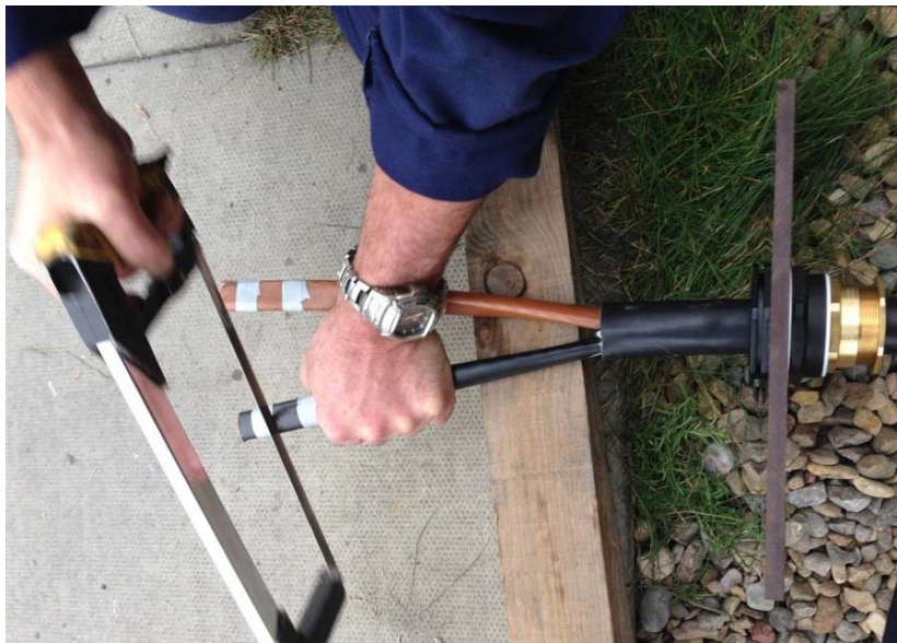
Figure 9: Cable cut to length
