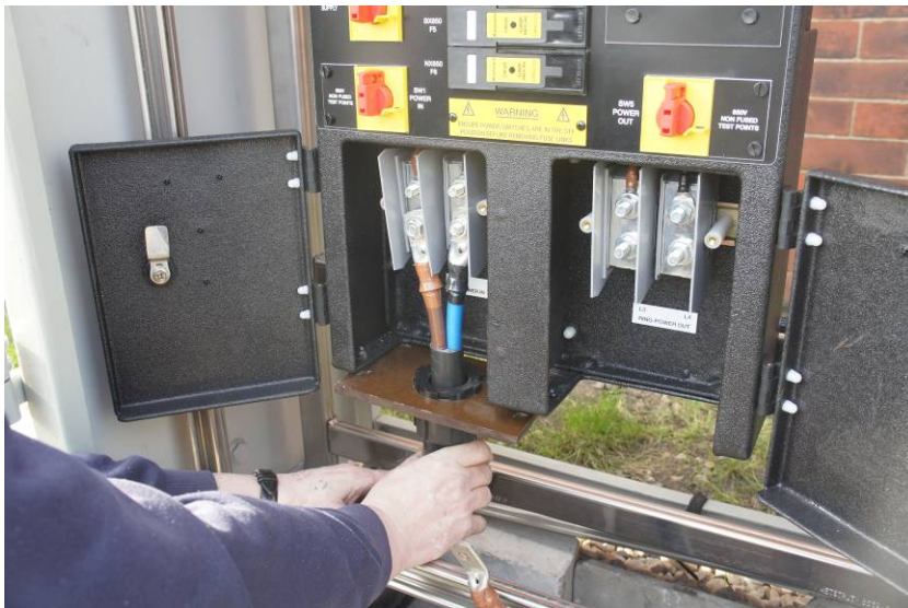
Figure 9: Refit Gland Plate
