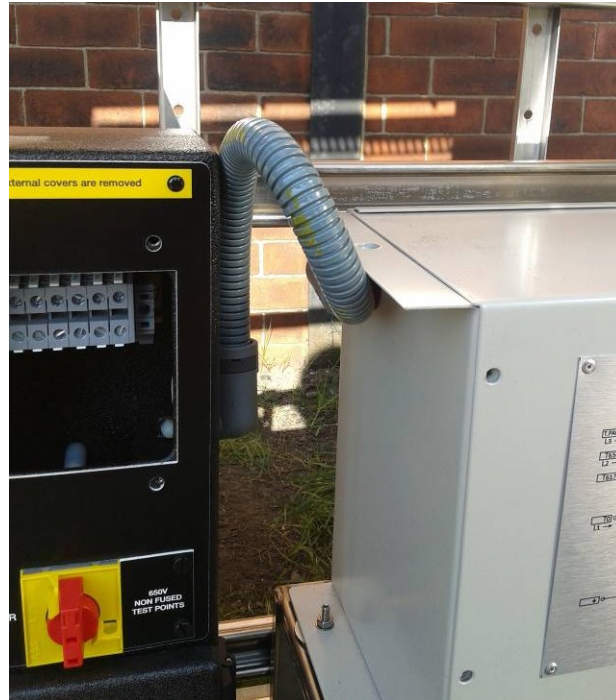
Figure 16: Transformer Conduit to SafeBox Installation
