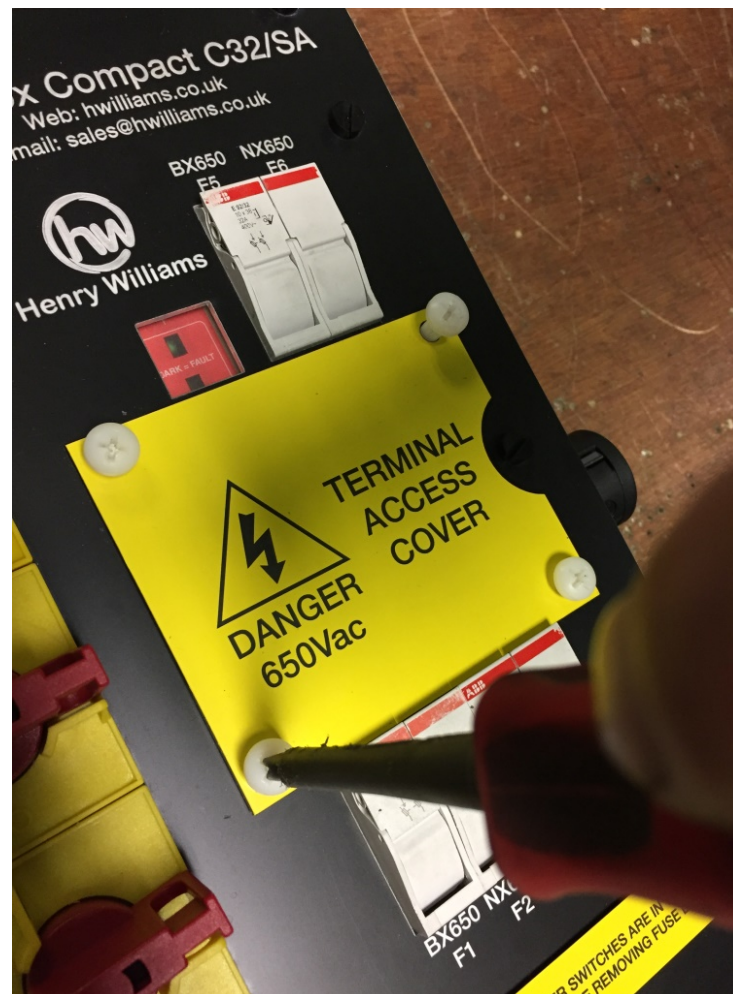
Figure 12: Removal of Terminal Cover
