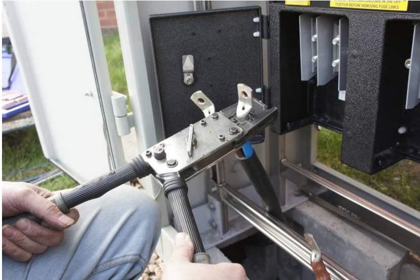
Figure 8: Fit & Crimp Cable Lugs
