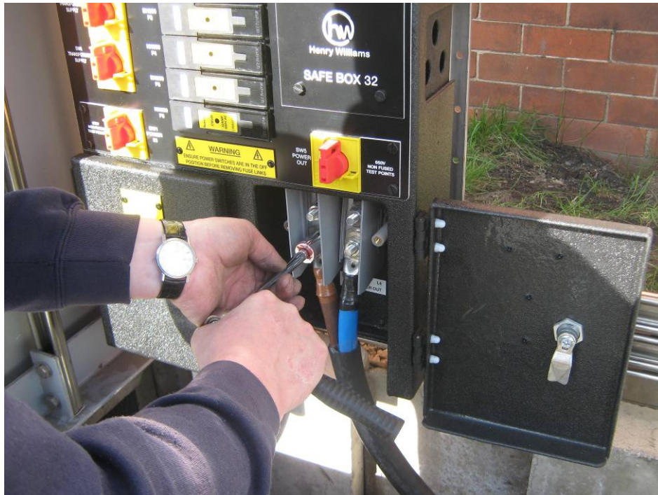
Figure 10: Complete Termination
