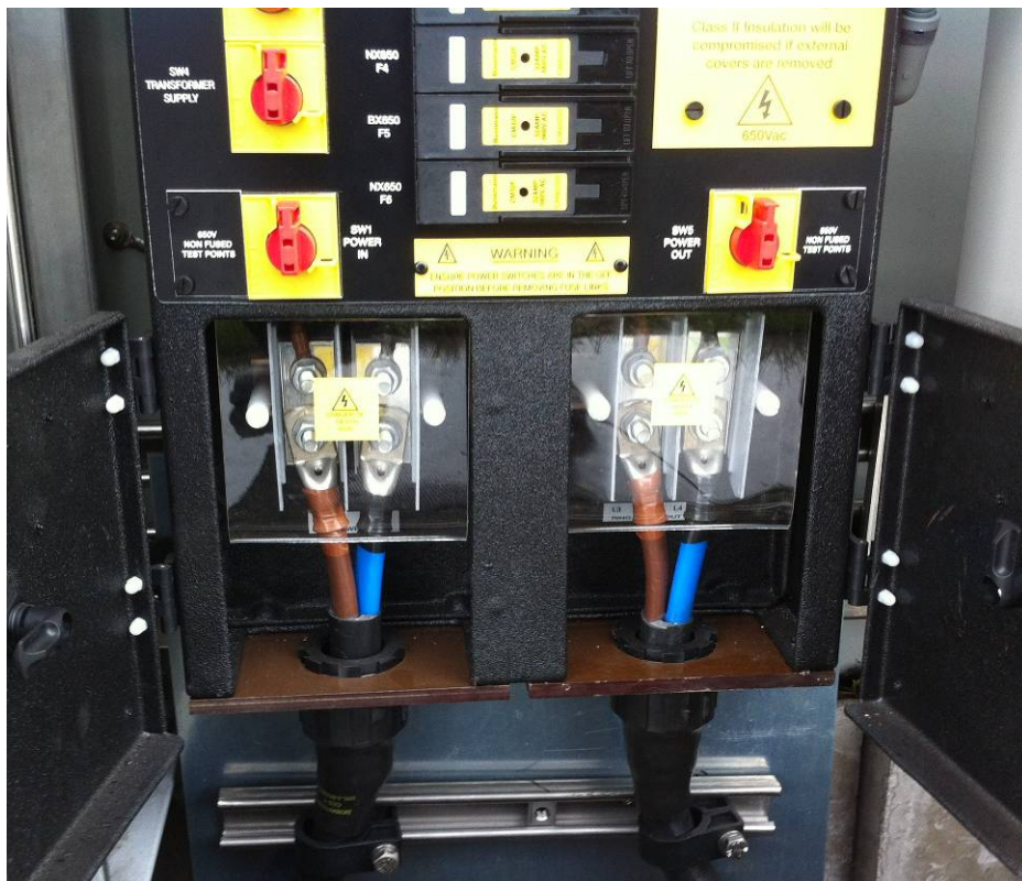
Figure 11: Refit Terminal Covers
