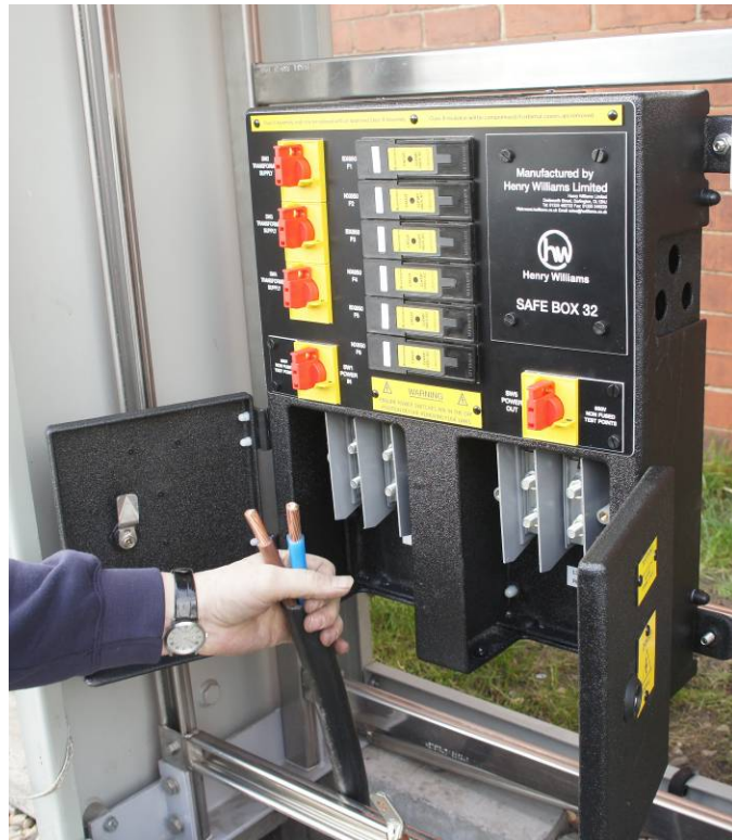
Figure 7: Cable cut to length
