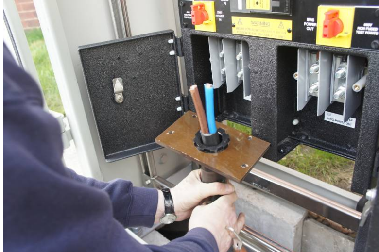
Figure 5: Cable Gland Plate removed from the enclosure
