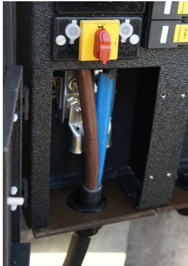
Figure 6: Cable length marked ready for cutting
