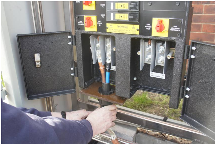
Figure 9: Refit Gland Plate
