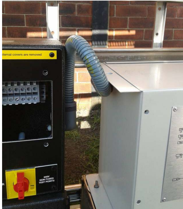
Figure 16: Transformer Conduit to SafeBox Installation
