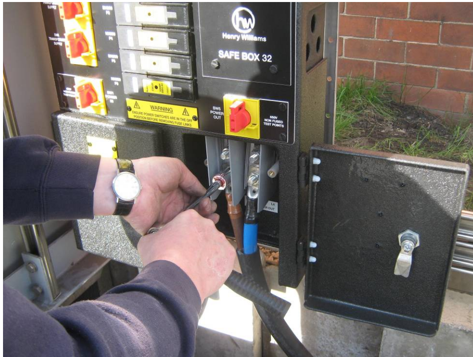
Figure 10: Complete Termination
