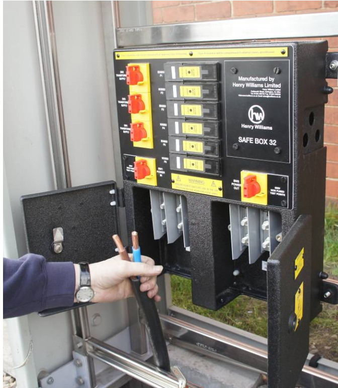
Figure 7: Cable cut to length
