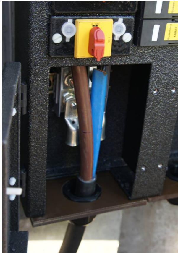
Figure 6: Cable length marked ready for cutting
