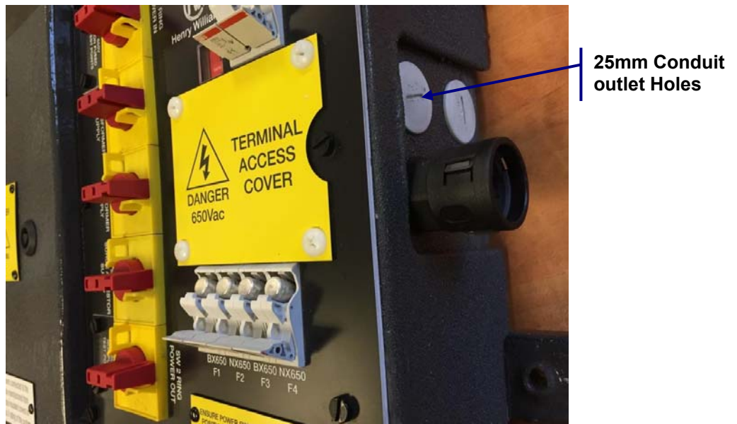
Figure 3: Functional Circuits/Transformer Wiring Outlets
