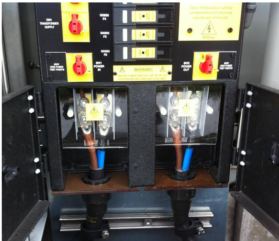
Figure 11: Refit Terminal Covers
