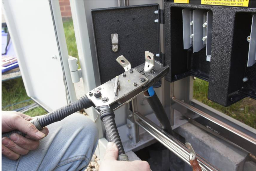
Figure 8: Fit & Crimp Cable Lugs
