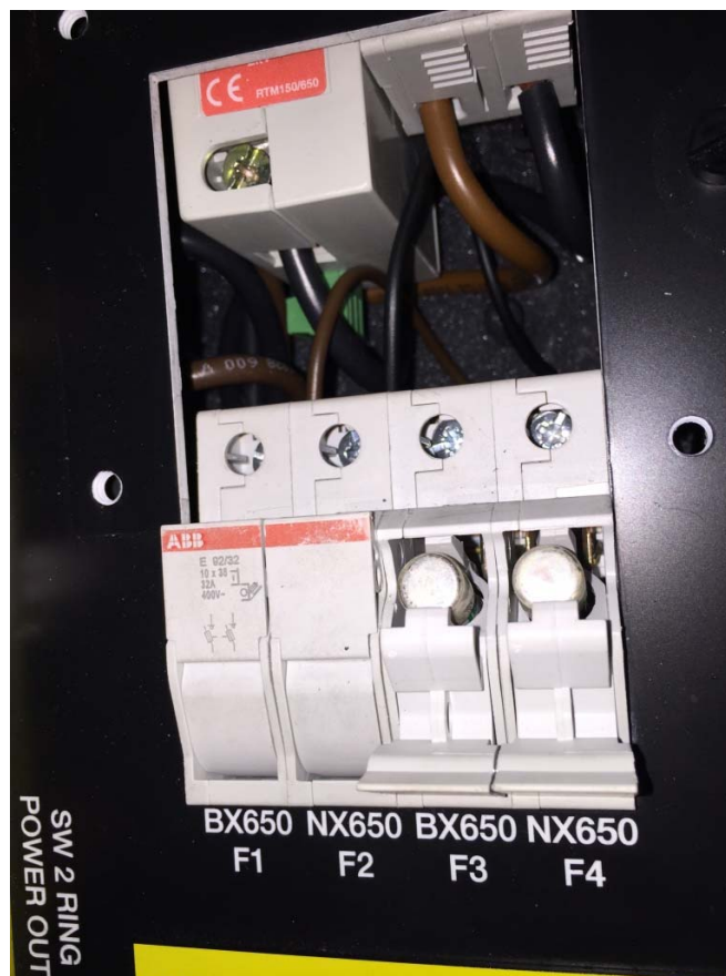
Figure 15: Functional Wiring Terminated
