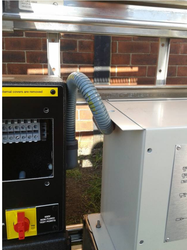
Figure 26: Transformer Conduit to SafeBox Installation
