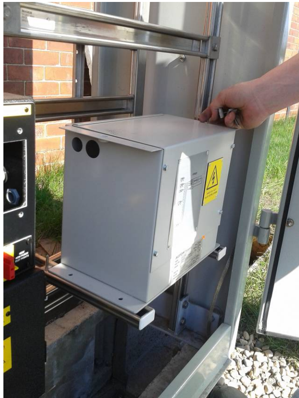
Figure 25: Transformer in Position
