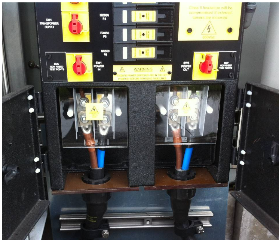
Figure 20: Refit Terminal Covers
