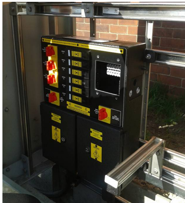
Figure 23: Terminal Cover Removed
