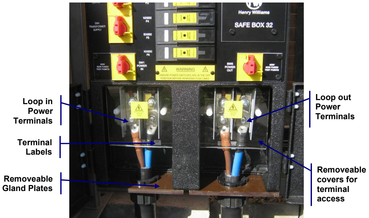
Figure 3: Power In/Out Terminal Arrangement
