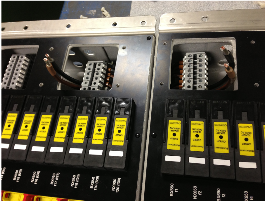
Figure 11: Wiring Tails fed through SafeBox Modules
