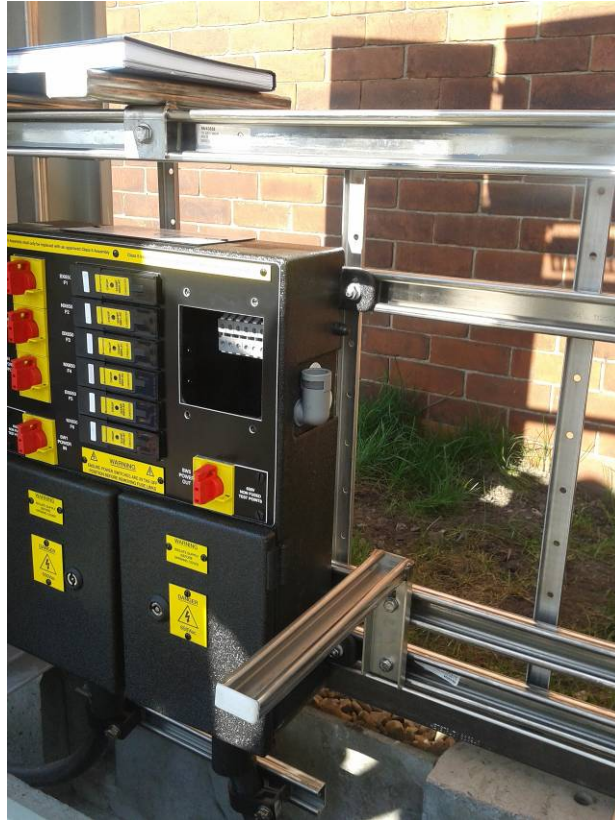
Figure 24: Glands & End Caps Applied
