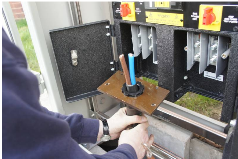
Figure 14: Cable Gland Plate removed from the enclosure
