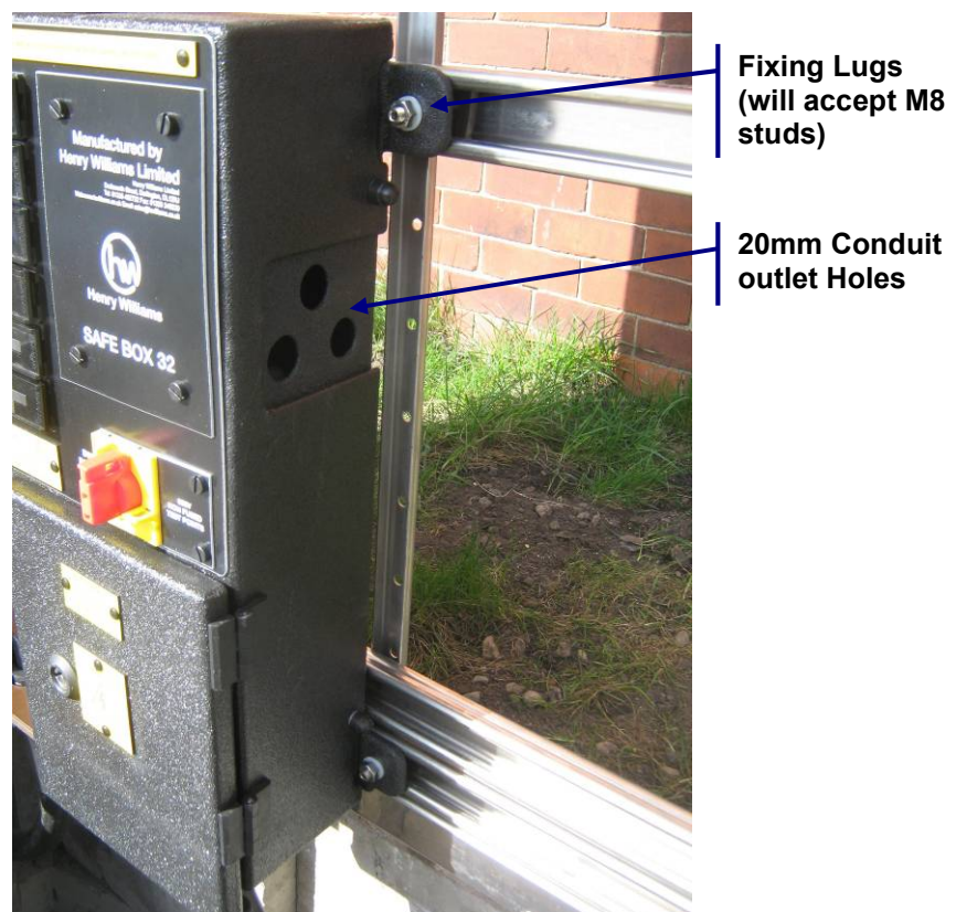
Figure 4: Transformer Wiring Outlets
