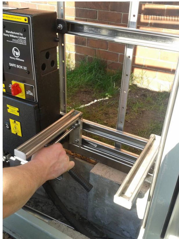
Figure 21: Assembly of BRS-SM440 Transformer Brackets
