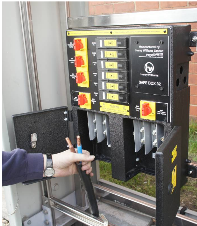
Figure 15: Cable length marked ready for cutting
