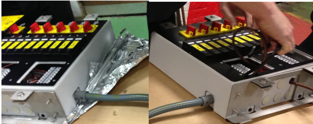
Figure 13: Conduit Location for Remote Connected SafeBox Modules
