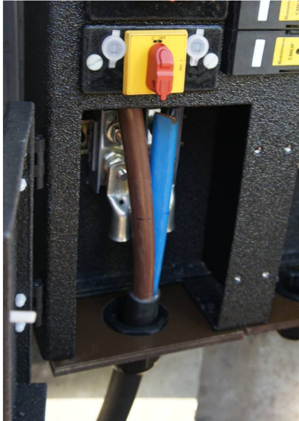
Figure 15: Cable length marked ready for cutting
