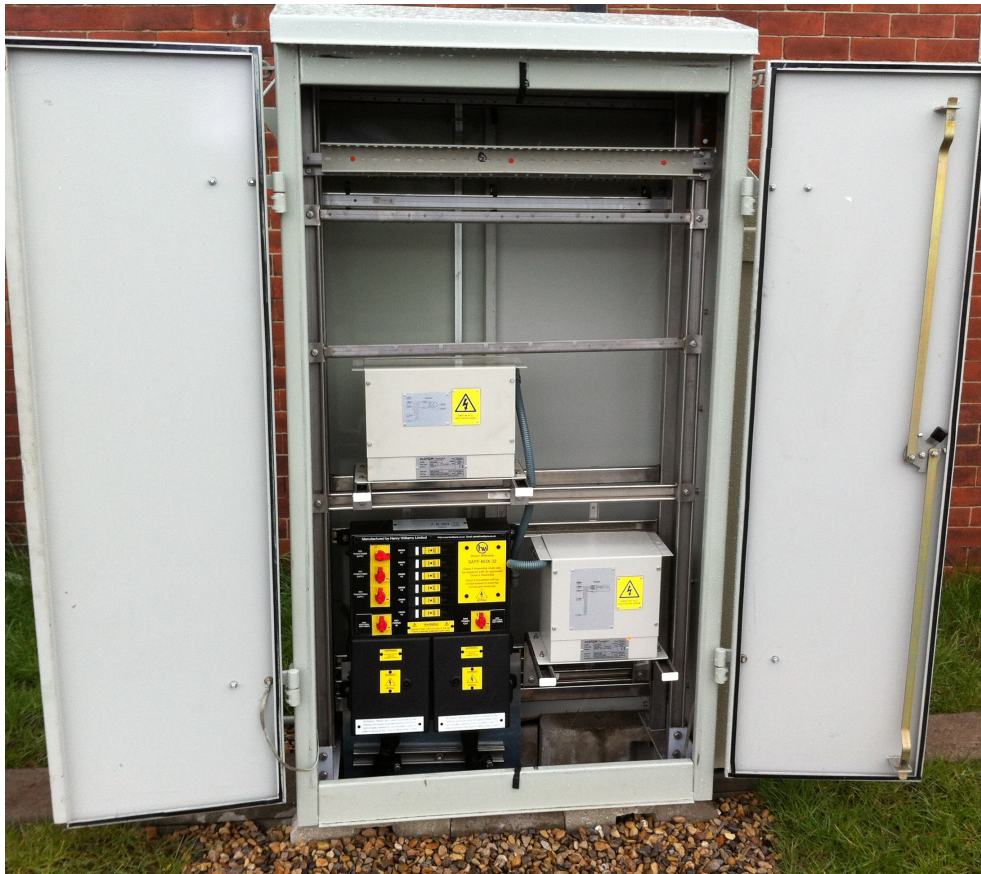
Figure 5: SafeBox installed into a Location Case
