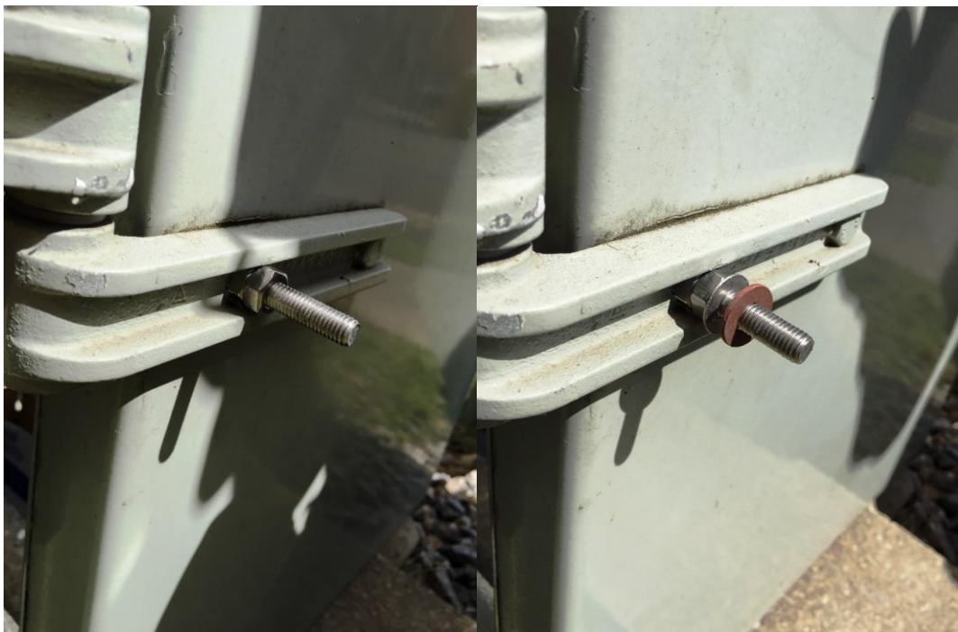
Figure 10: Two plain M8 nuts followed by plain and vulcanised washer
