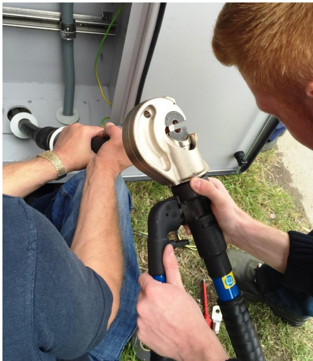
Figure 17: Use of Cable Rounding Die in Crimp Tool
