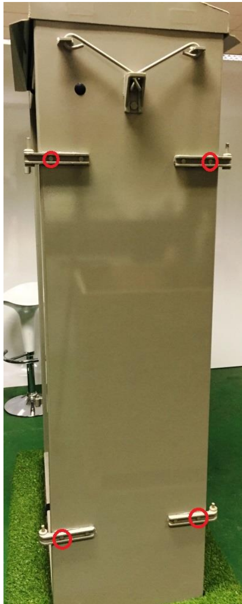
Figure 4: Location Case Hinge Bolt Positions
