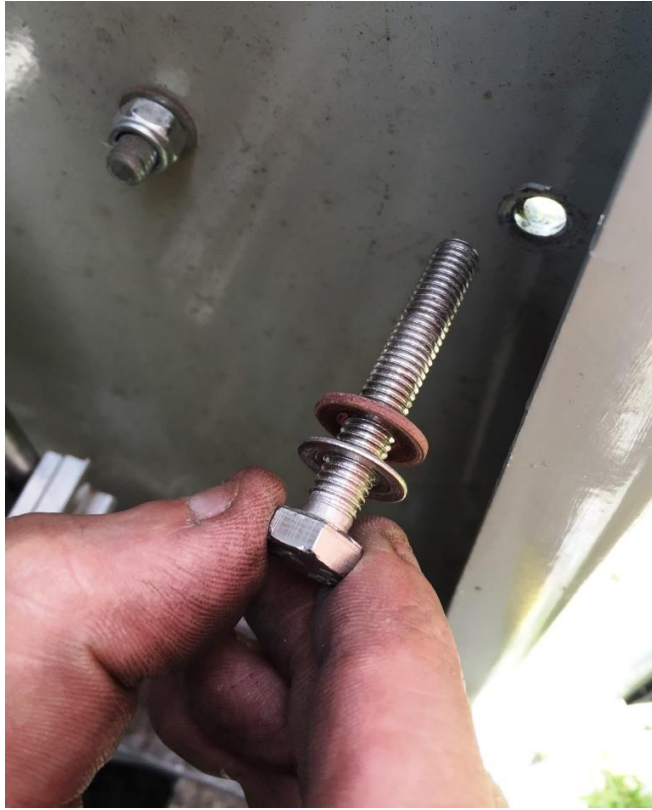
Figure 9: Plain and vulcanised washers on M8 x 50 bolt
