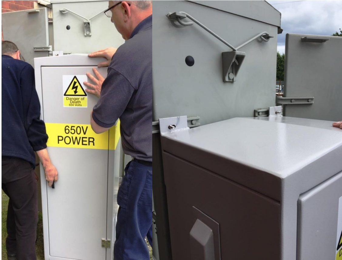
Figure 11: Lift enclosure into position onto the protruding bolts
