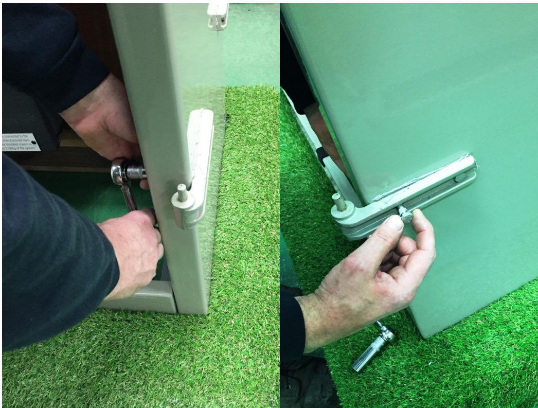
Figure 8: Remove existing outer door hinge bolts
