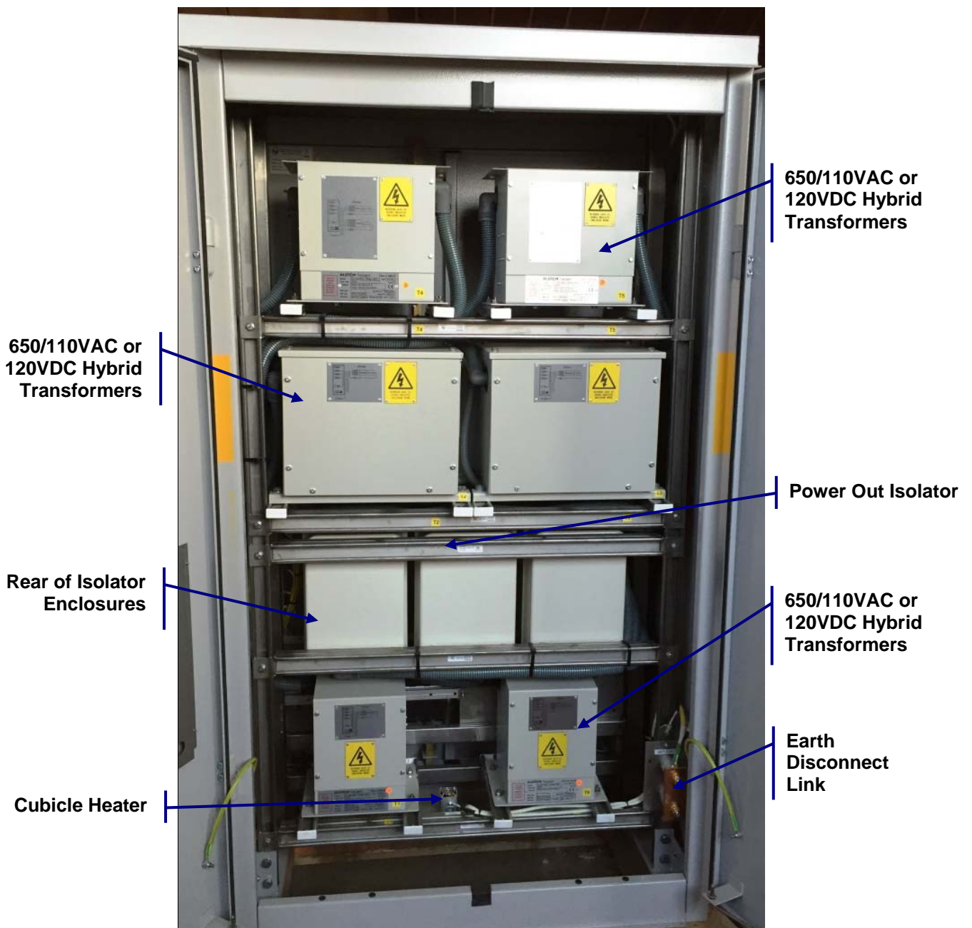
Figure 8: FSP01/02 (Loc + power) Front Arrangement
