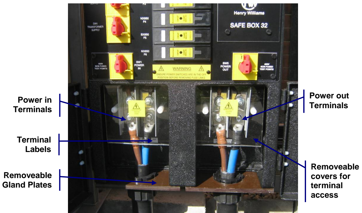
Figure 13: Power In/Out Terminal Arrangement
