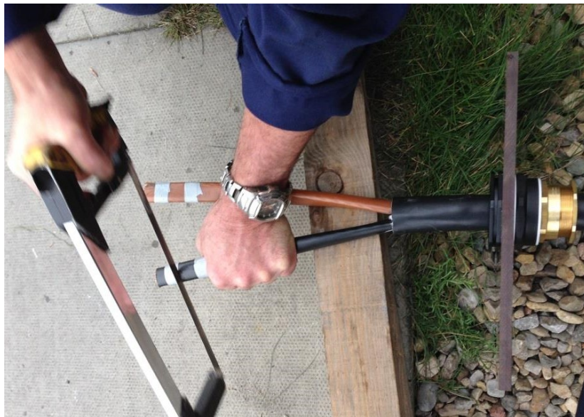
Figure 11: Cable cut to length
