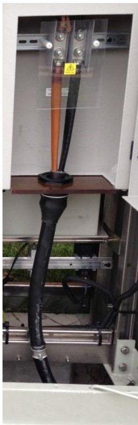
Figure 16: Final installation of terminated cables
