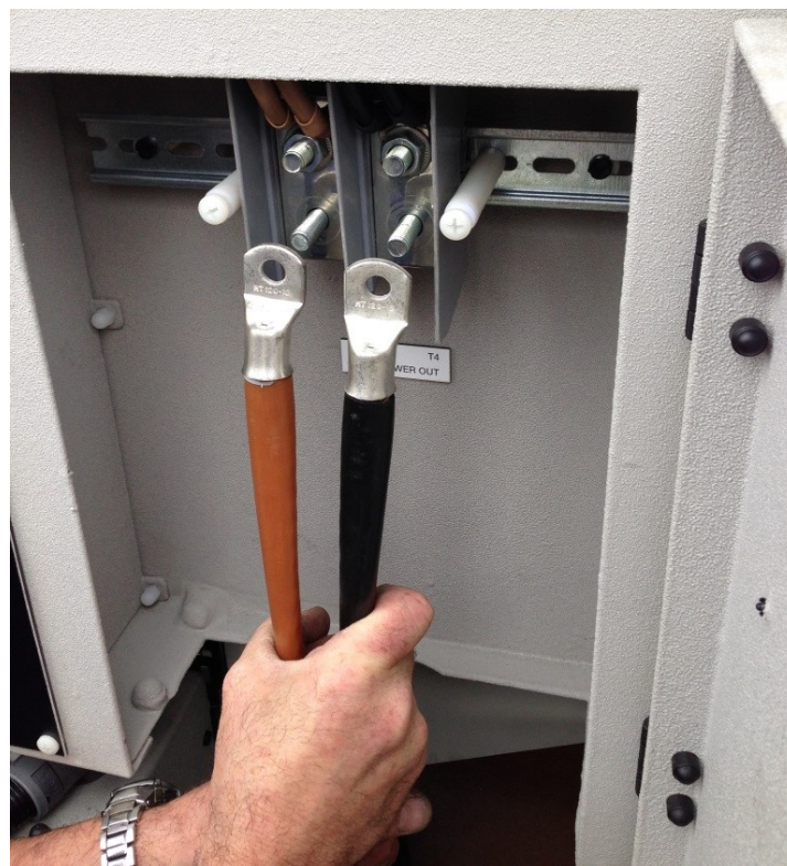
Figure 13: Orientation of crimp lugs with the terminal studs
