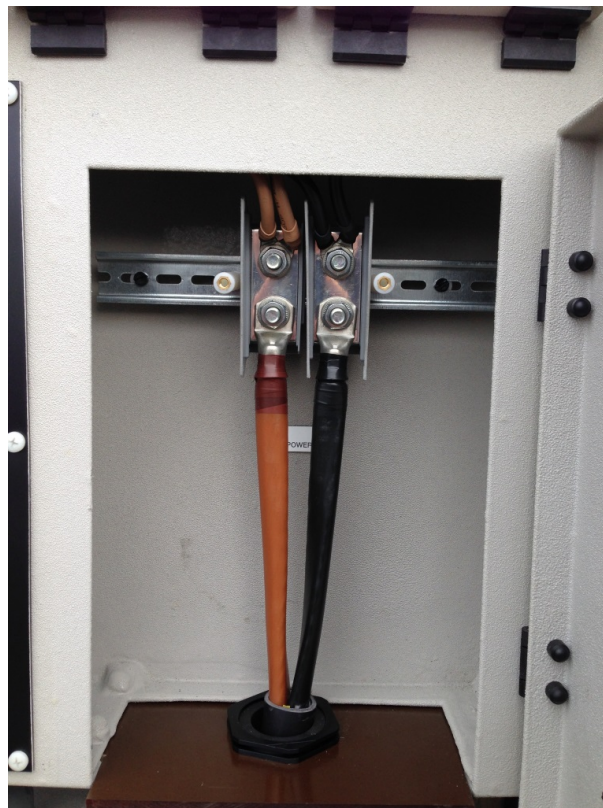
Figure 15: Tape crimps & terminate cable
