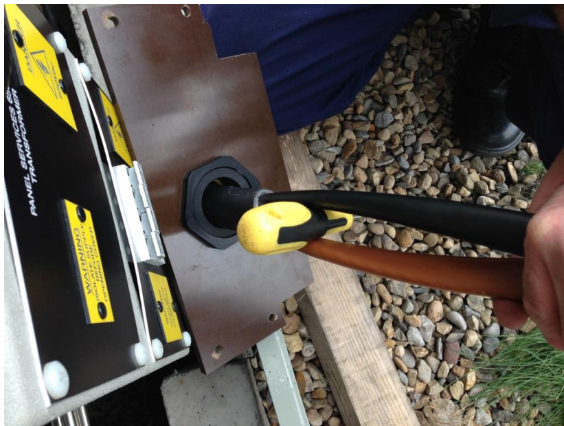
Figure 9: Forming Cable V shape
