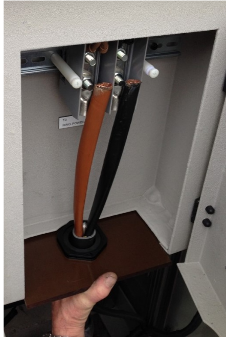
Figure 10: Cable length marked ready for cutting
