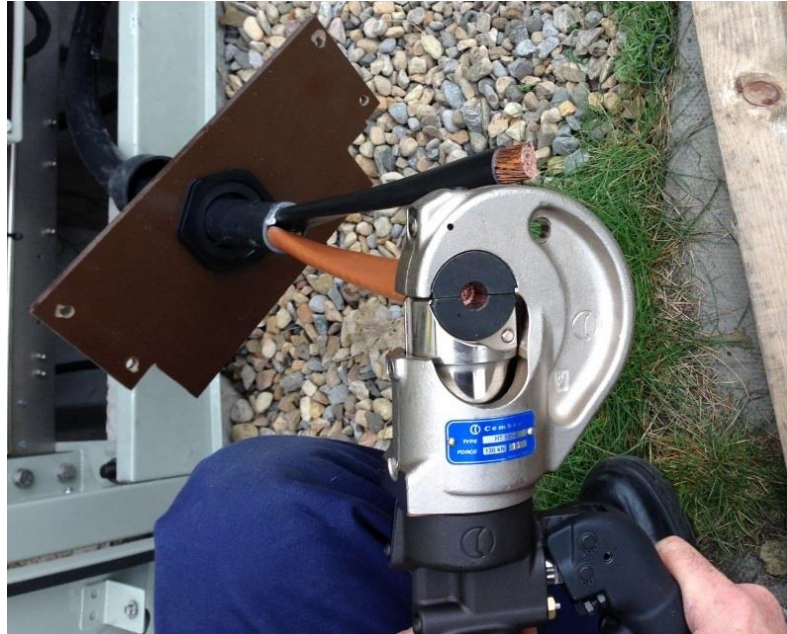
Figure 12: Rounding Cable ends using tool
