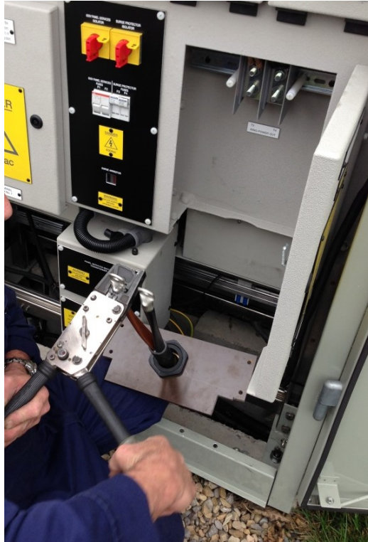
Figure 14: Crimping Cable Lugs
