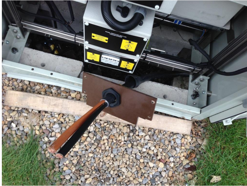
Figure 8: Installed Cable into removed Gland Plate
