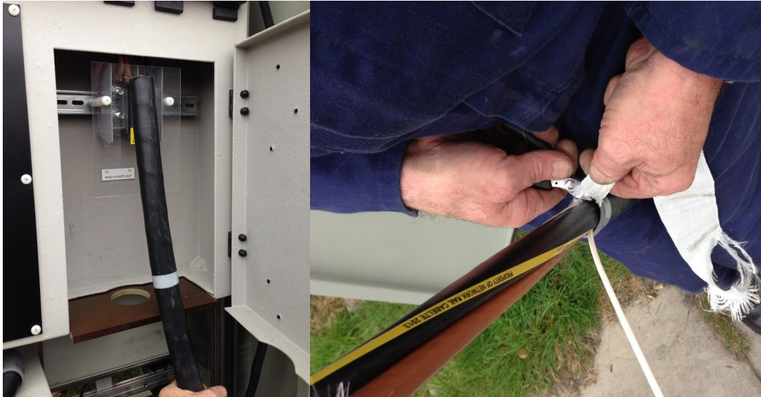
Figure 6: Measure & Strip Cable
