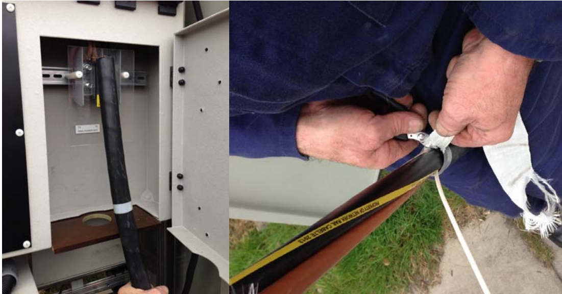
Figure 6: Measure & Strip Cable
