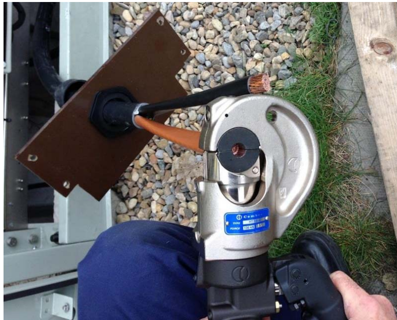
Figure 12: Rounding Cable ends using tool
