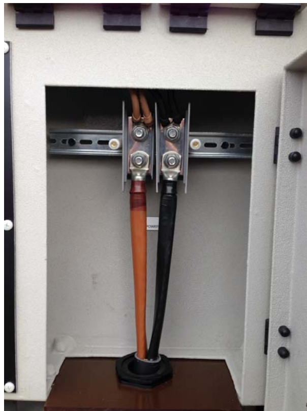
Figure 15: Tape crimps & terminate cable
