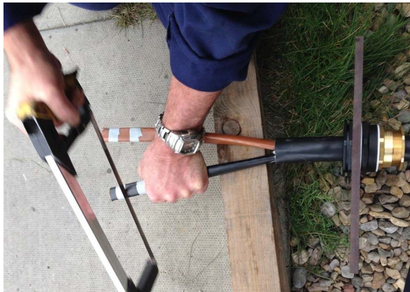
Figure 11: Cable cut to length
