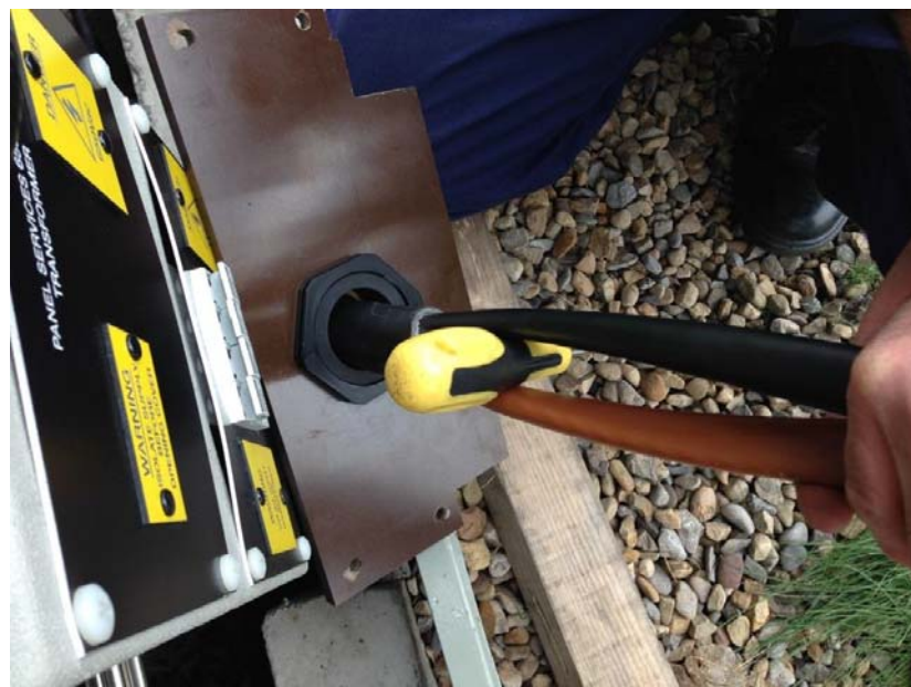
Figure 9: Forming Cable V shape
