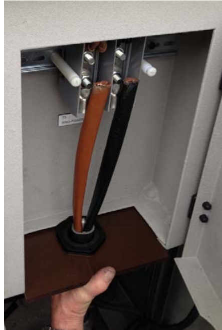
Figure 10: Cable length marked ready for cutting
