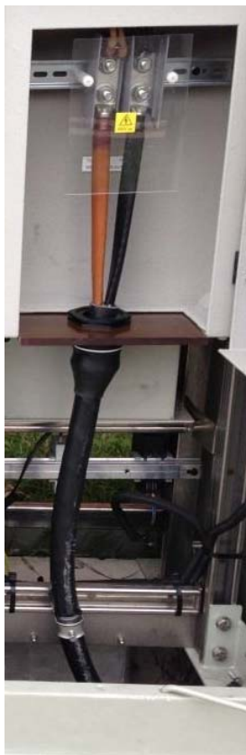
Figure 16: Final installation of terminated cables
