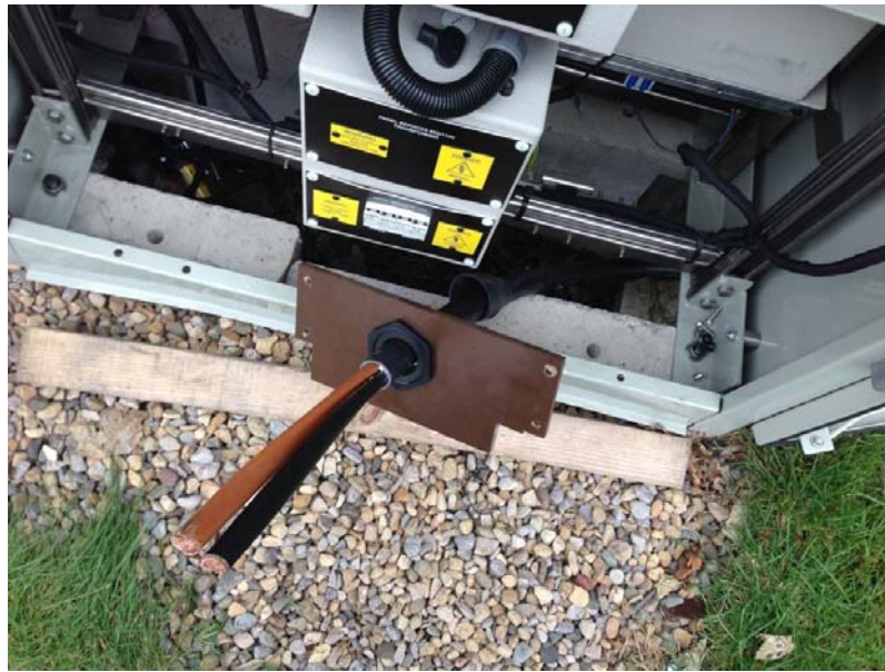
Figure 8: Installed Cable into removed Gland Plate
