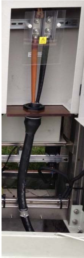
Figure 16: Final installation of terminated cables
