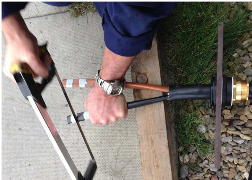
Figure 11: Cable cut to length
