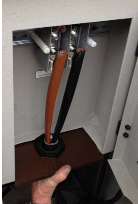
Figure 10: Cable length marked ready for cutting
