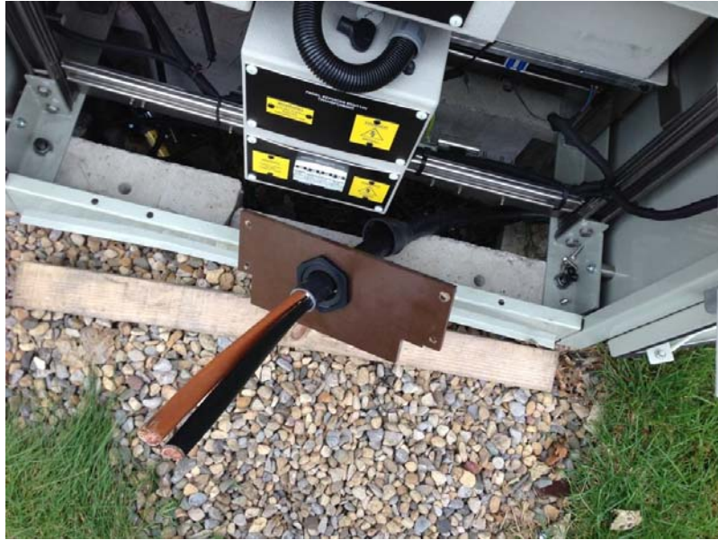
Figure 8: Installed Cable into removed Gland Plate
