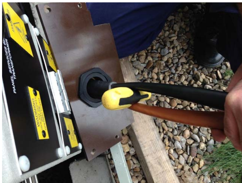
Figure 9: Forming Cable V shape
