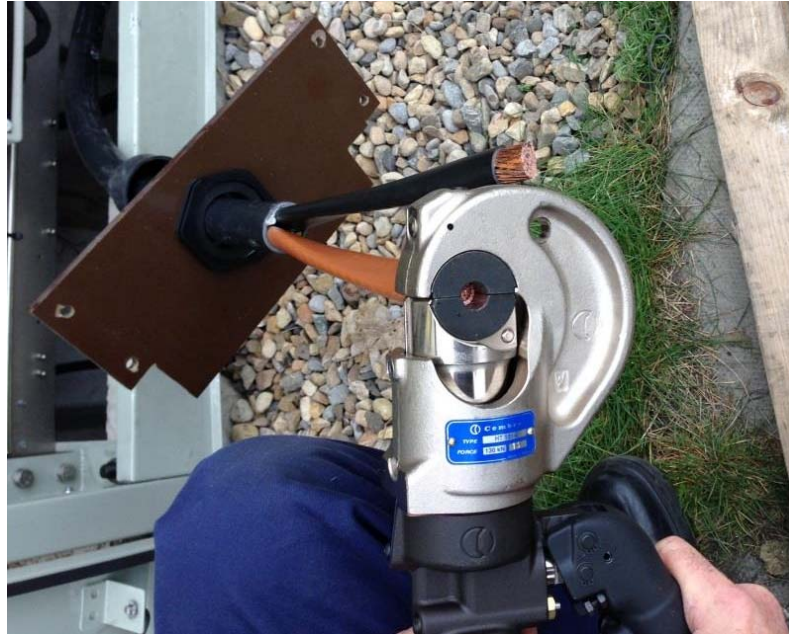
Figure 12: Rounding Cable ends using tool
