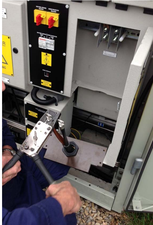
Figure 14: Crimping Cable Lugs
