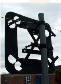
Signal frames are manufactured from aluminium then powder coated black in accordance with TR2180 and are designed to MCX0043, MCX0202 and MCX 201 Highways Agency specifications for mounting matrix signs and lanterns on:-
