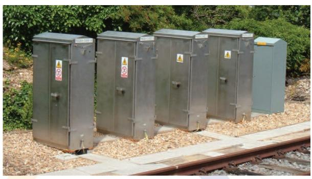
IN terms of securely housing safety-critical trackside communication equipment and switchgear, the right location case is everything.
